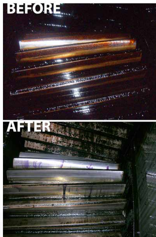
Above: A ball mill pinion gear is coated with a thick accumulation of asphaltic open gear lubricant. Below: After conversion to LE's Pyroshield synthetic lubricant, the pinion is clean.
